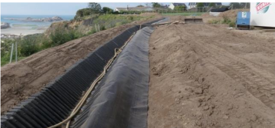
Installation with lateral flow edge protection
