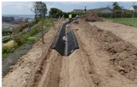
SmartDitch being installed on the crest to catch runoff
