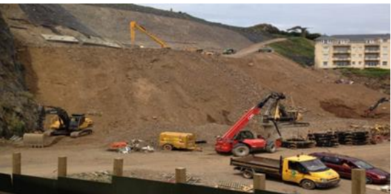
View from the bottom of the quarry during construction
