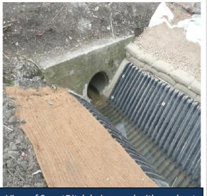
View of SmartDitch being used with a culvert
