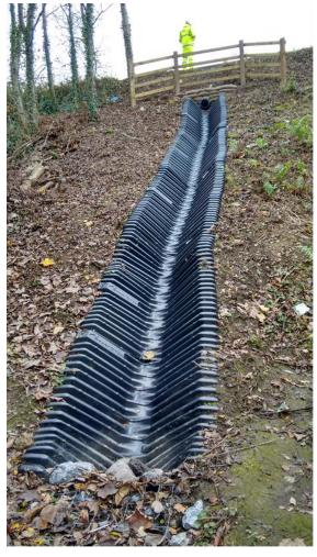
steep embankment (1:1.5). The solution included a shallow 225 outfall diameter mm pipe, connected to 10 а m long SmartDitch section laid on the embankment. At the bottom end of the chute, a gabion basket was installed for energy dissipation before the water reaches the river. Concrete was only used for the bagwork headwall of the outfall pipe.
