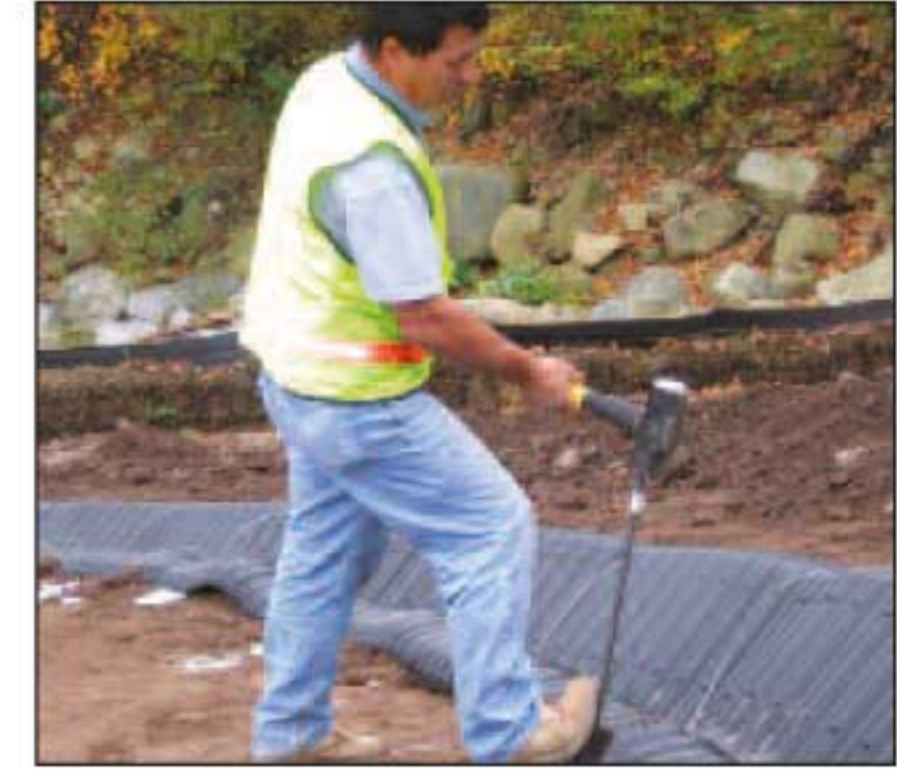
The SmartDitch anchoring system installs quickly and secures the system into the ground.
