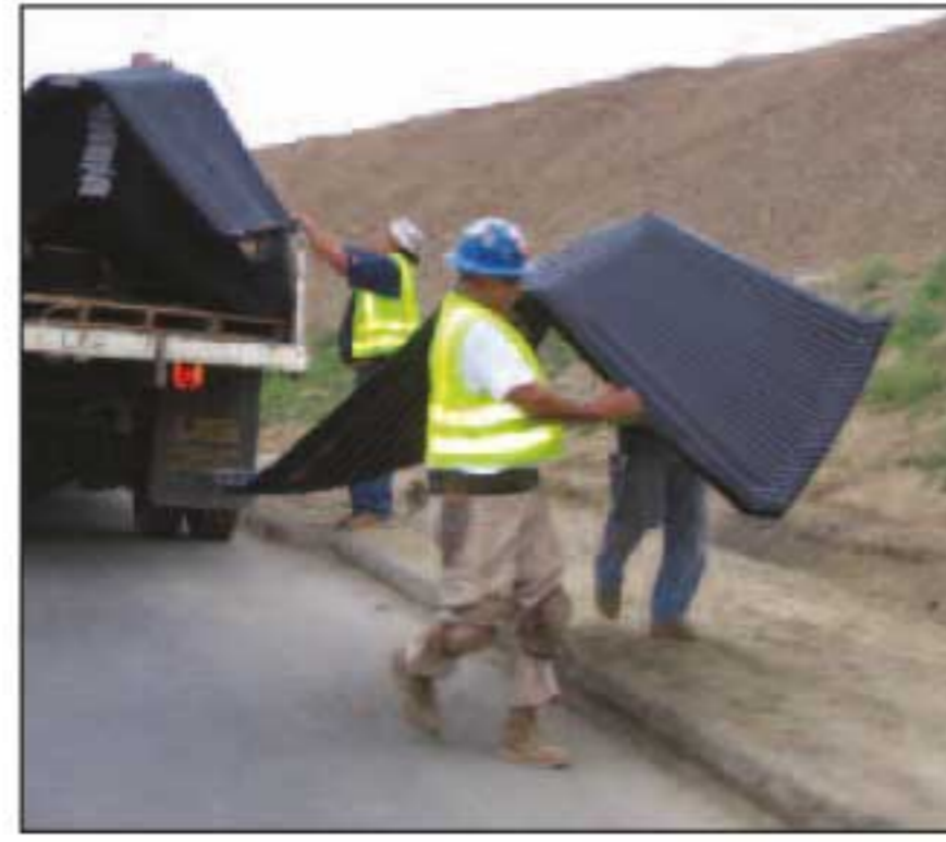
SmartDitch is light enough to be hand-carried to the trench, and allows for easy transport to areas where vehicle access is limited.
