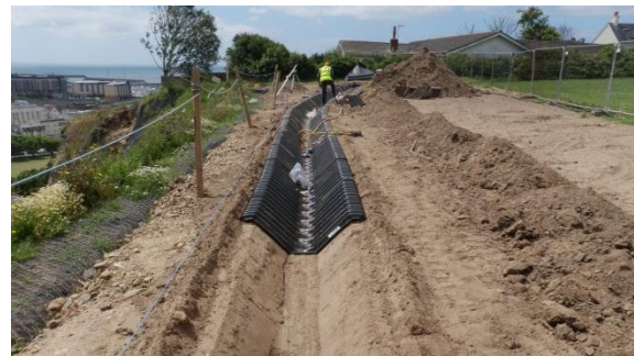
SmartDitch being installed on the crest to catch runoff
