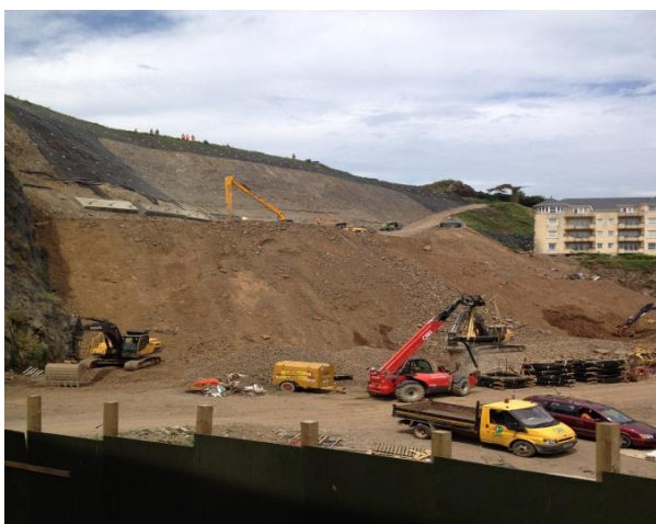
View from the bottom of the quarry during construction
