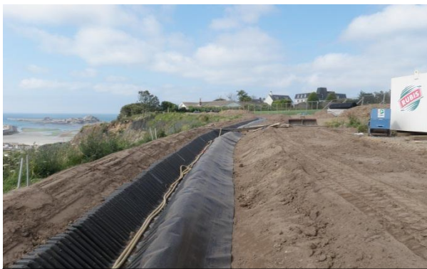
Installation with lateral flow edge protection
