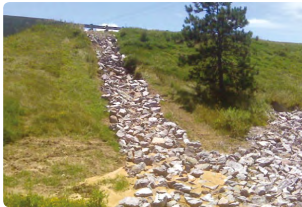
Portage, WI Before: Riprap continued to fail at this DOT drainage outfall.
