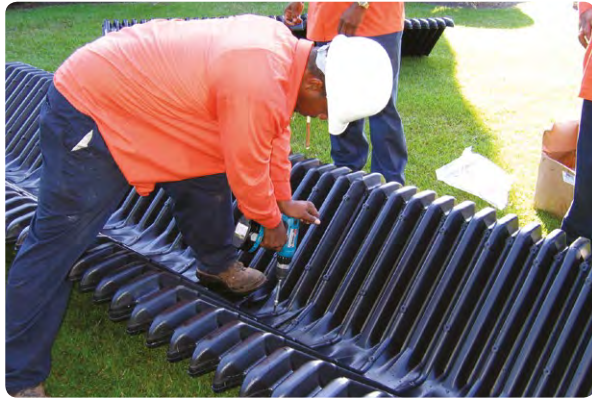
Self-tapping screws hold the channel together.
