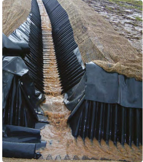
Edge protection prevents soil erosion from lateral flow.
