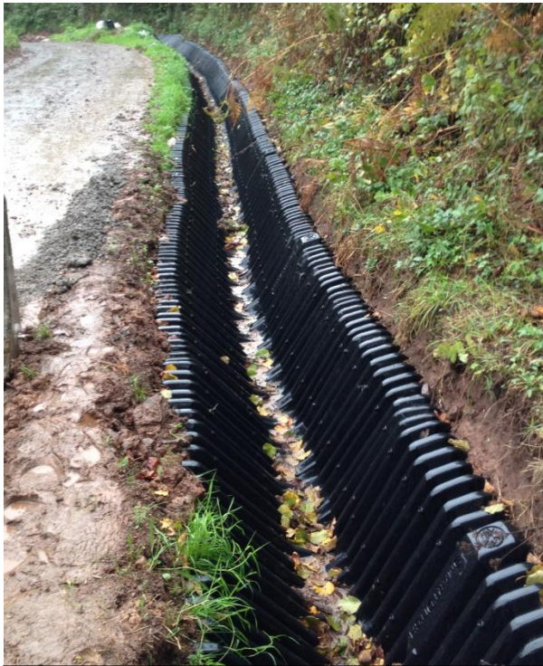
SmartDitch Installed along the side of the road
