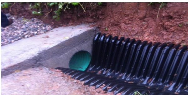
SmartDitch is sealed against the concrete face
